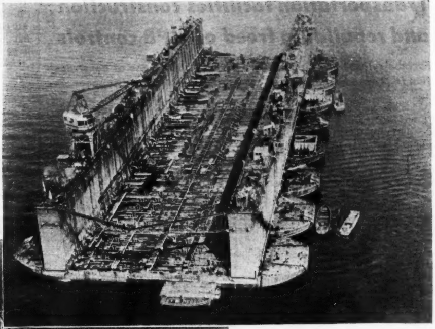
Drydock above is shown in raised position with keel and bilge blocks set to accommodate a ship.
